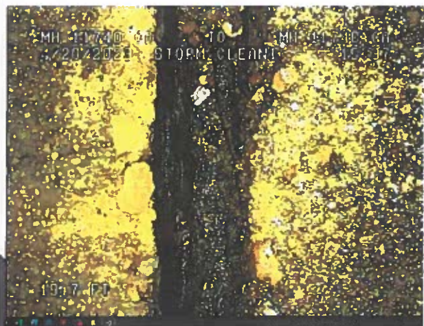
Examples of Joint Separation
