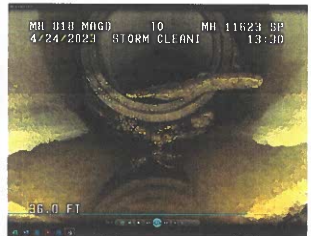
Examples of Vertical Misalignment
