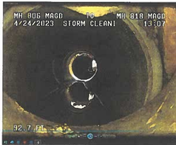
Examples of Vertical Misalignment
